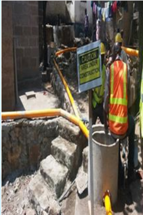
Construction of Simplified Sewerage system (condominal system) in Mwanza
